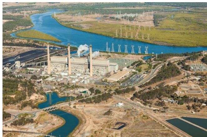
Figure 3.13: The Gladstone coal-fired power station, on the bank of the Calliope Estuary, from the north-east.
