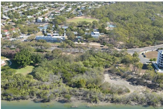
Figure 16. Flood damaged shoreline vegetation - Boyne River estuary, Zone 10.
