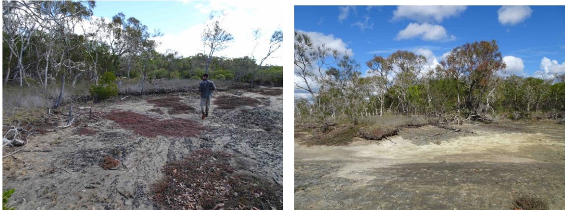
Figure 18A & B. Retreat and erosion of the terrestrial fringe is a serious growing threat to supra-tidal habitats throughout the study area—Colosseum Creek, Zone 11a.
