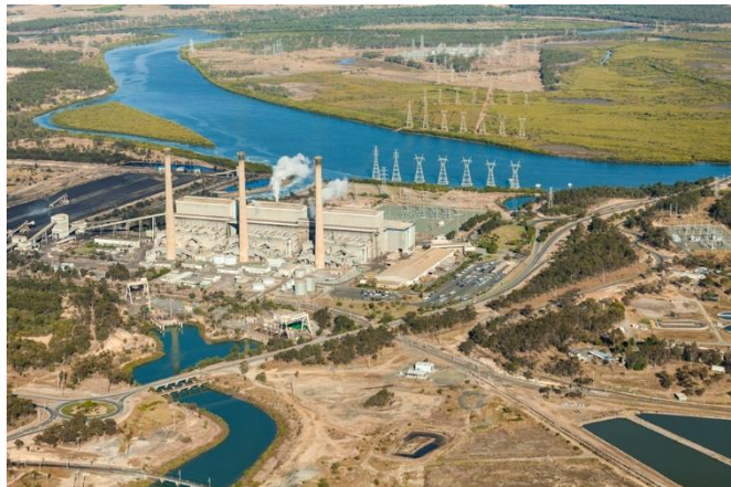
Figure 7.13: The Gladstone coal-fired power station, on the banks of the Calliope Estuary photographed from the north-east.
