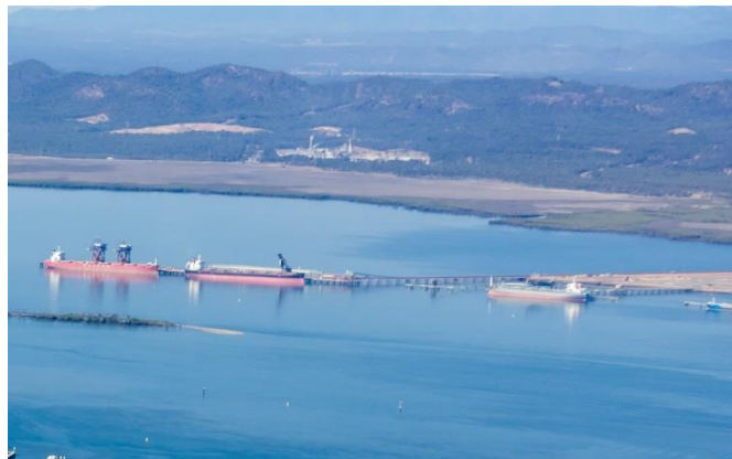
Figure 7.9: Inlet to Boat Creek photographed from the Western Basin.
