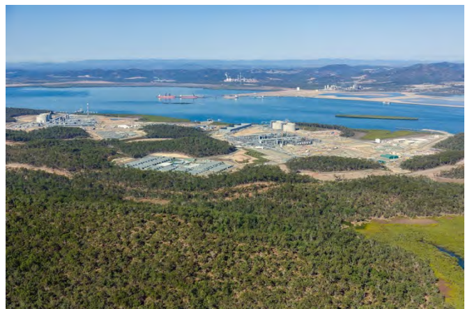
Figure 10.7: The south-western corner of Curtis Island, showing two LNG plants in the foreground and the Western Basin in the distance.
