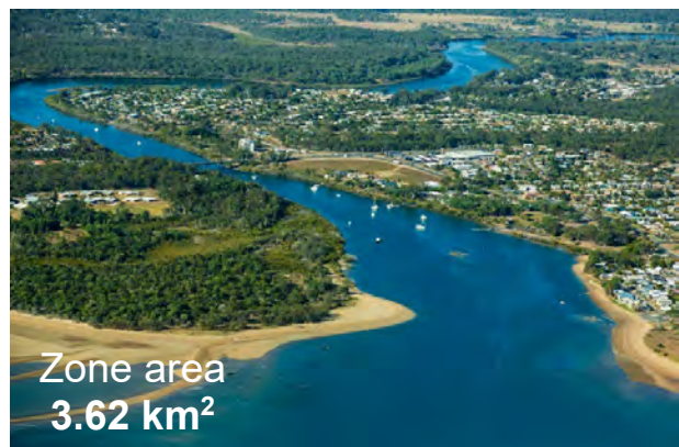
Figure 10.21 | The mouth of the Boyne River photographed from the north-east. Boyne Island is on the right and Tannum Sands on the left.
