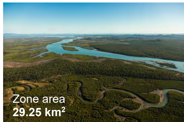
Figure 10.3 | The Narrows photographed from the south with Keppel Bay in the distance.
