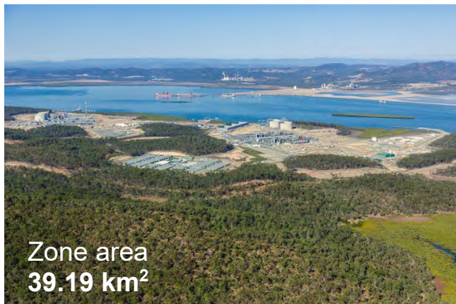
Figure 10.7 | The south-western corner of Curtis Island, showing two liquid nitrogen gas plants in the foreground and the Western Basin in the distance.
